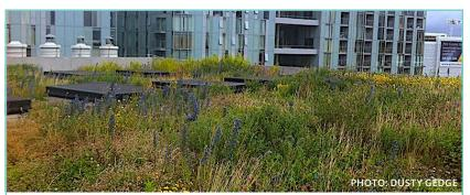
**Extensive roof.** Extensive roofs are lightweight systems and typically include drought tolerant self-seeding sedums, grasses, mosses and meadow flowers requiring little or no irrigation (dependent on the regional climate) and less maintenance after establishment. These roofs are not intended for recreation, or to accommodate the weight of people, larger shrubs or trees (Green Plants for Green Buildings, 2014).
