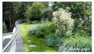
*Intensive roof.* Intensive roofs can be thought of as a rooftop garden where anything is possible if you have the weight bearing capacity. Trees, shrubs and water features may be installed and provide access for people.
